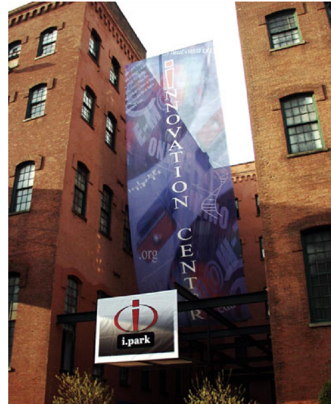
i.park Hudson at 28 Wells Avenue, Yonkers
